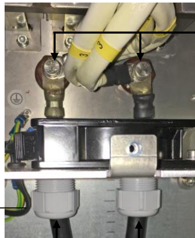
Fig. 7: Connection Track Cable
